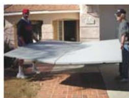
Transport Pads to Location
