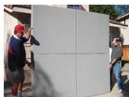
Lift Up Assembled Pads
